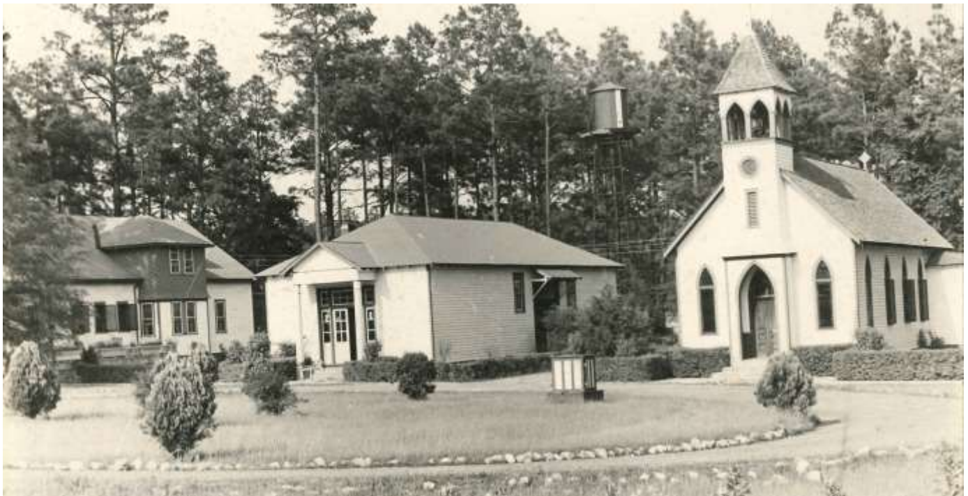
MINE CREEK, WARD, SC
